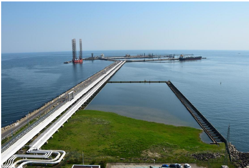
Pic. 6 View of new quay location
