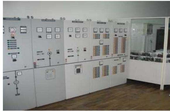
Figure 1 Main switch board
